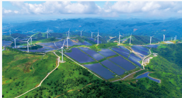
Photovoltaic Power Business in Yeongam
